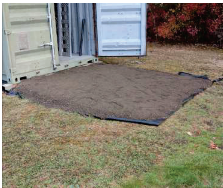
Gravel ramp in progress. As discussed in the October meeting, this will make moving the mowers easier and safer.
